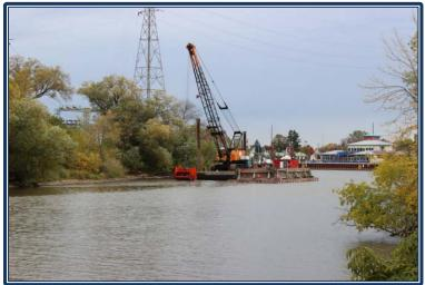
Figure 4 - River dredging with crane barge and material scow
